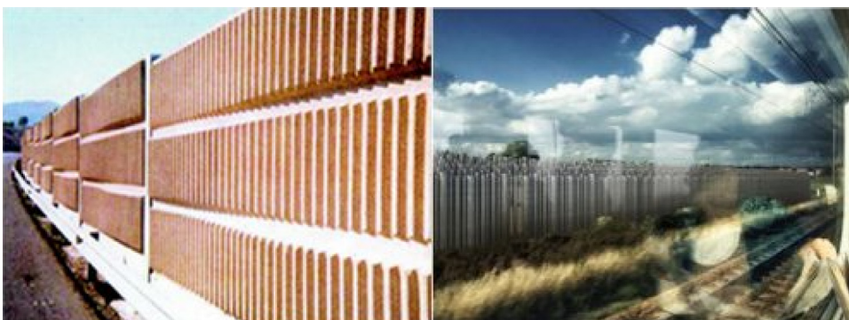
FIG. 6. (Color online) (a) Picture of a conventional acoustic barrier. (b) Simulated acoustic barrier based on SC.
